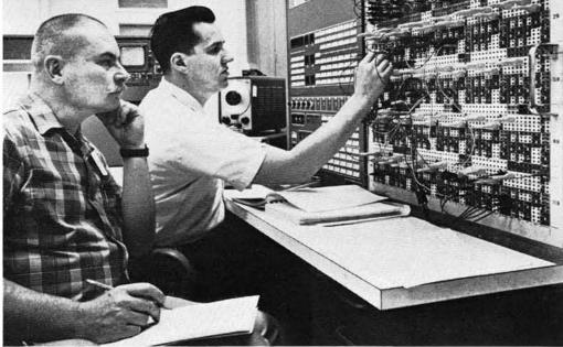
JIM ALLENSWORTH (left) and Ron Domres (both 9422) are at the EAI-680 console with the patch panel in position. In the background are sine-wave generator, oscilloscope, and plotter.
